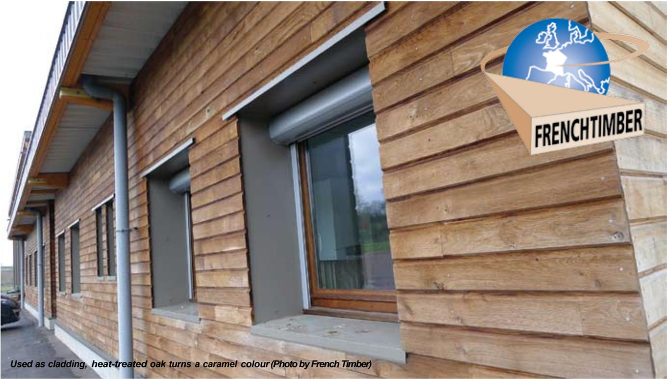
Used as cladding, heat-treated oak turns a caramel colour (Photo by French Timber)
